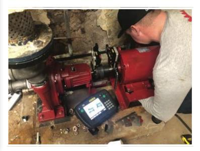
Correct shaft alignment ensures the smooth, efficient transmission of power from the motor to the pump. Incorrect alignment occurs when the centerlines of the motor and the pump shafts are not in line with each other. Misalignment produces excessive vibration, noise, coupling and bearing temperature increases, and premature bearing, coupling or shaft failure.
